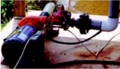
ABOVE: 2" Cycle Stop installed at Roseland Vineyard, Crozet, VA
